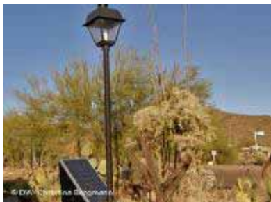
Solar collectors can be used for many purposes. Here they provide the light for the parking area of the Arizona-Sonora Desert Museum
